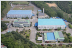
Cheonan factory (Korea) PLC, AC drive, HMI, DCS, PV module
