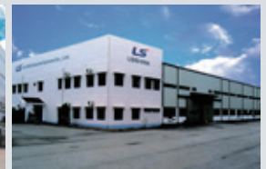
Hanoi factory (Vietnam) MV/LV switchgear, Mold TR
